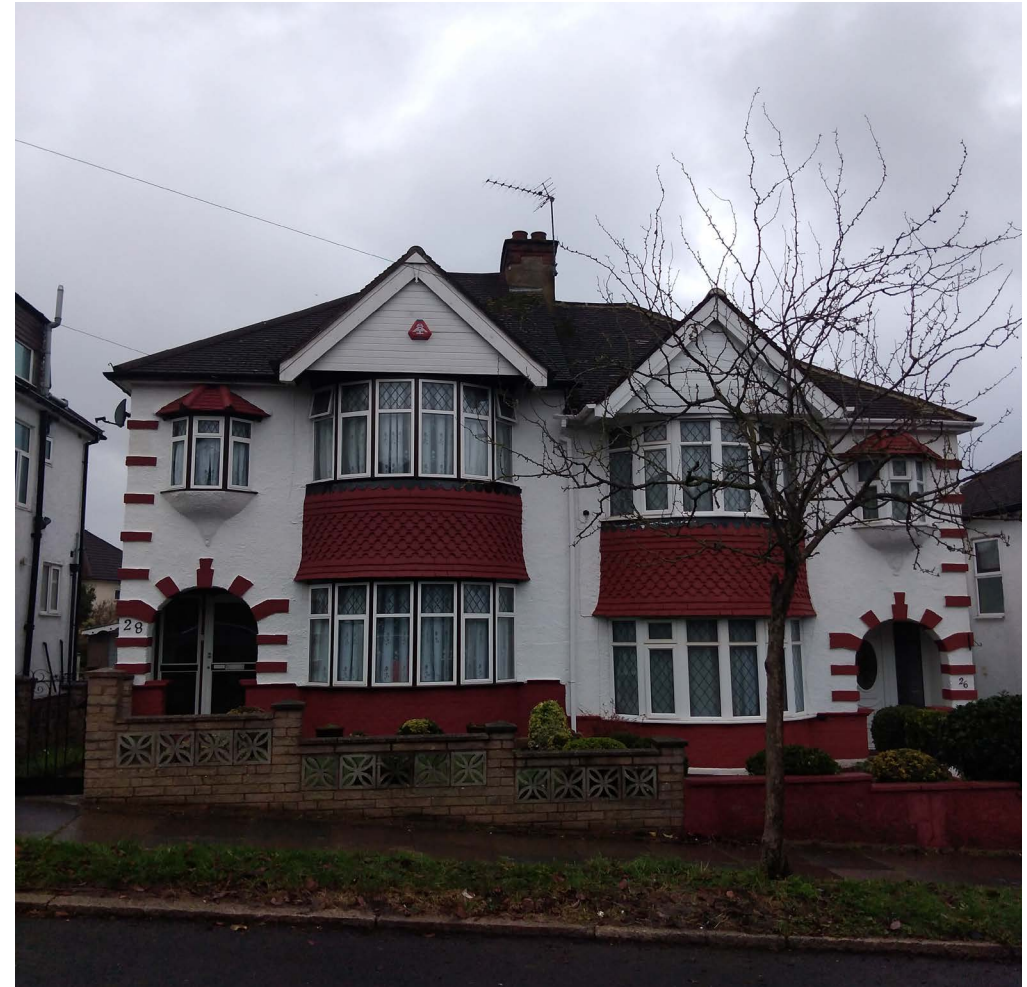
Figure 12: Houses on Buck Lane
