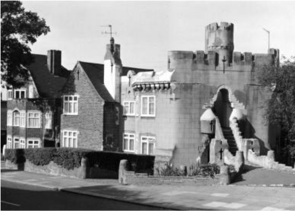
Figure 9: Highfort Court (1937) by Trobridge
